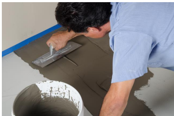
Trowel applied (flash) patch being applied
