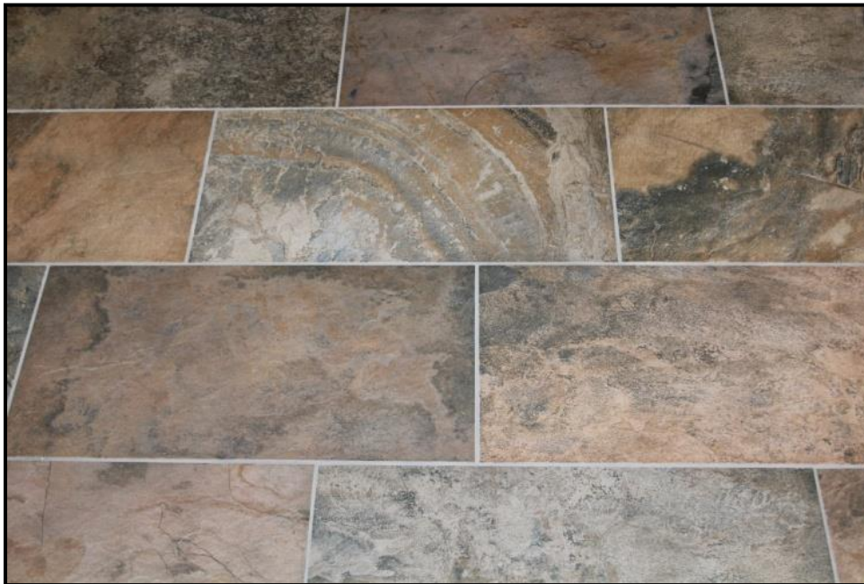
12' X 24" rectified porcelain tile installed using a 33% offset grout joint
