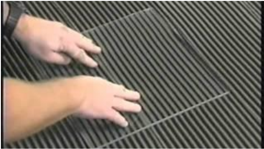
Straight troweling eliminates trapped air
